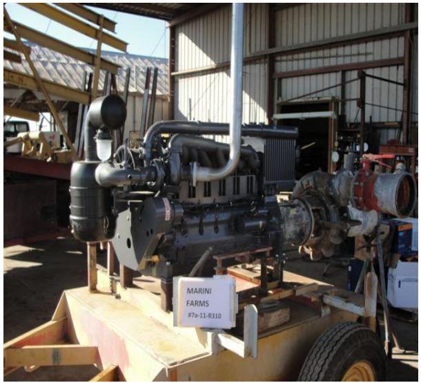
Marioni Project #2 (New Engine)
